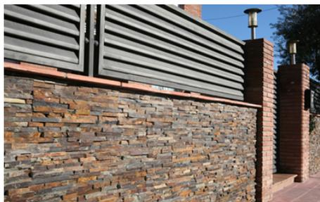
Culture Stone is manufactured to resemble the Natural Stone Veneer by using light weight concrete and a variation of color pigments and rubber or fiberglass molds. Another difference between the two types of veneers is the quality. It is important to choose a credible manufacturer of Culture Stone that can guarantee the quality of their product. With Natural Stone you do not have to worry about your material fading years after installed.
